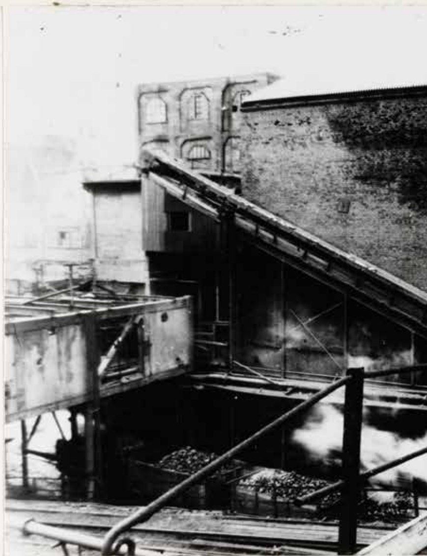
427 1200 TON BUNKER WITH ELEVATOR DRIVE ON AXIAL ON TOP
